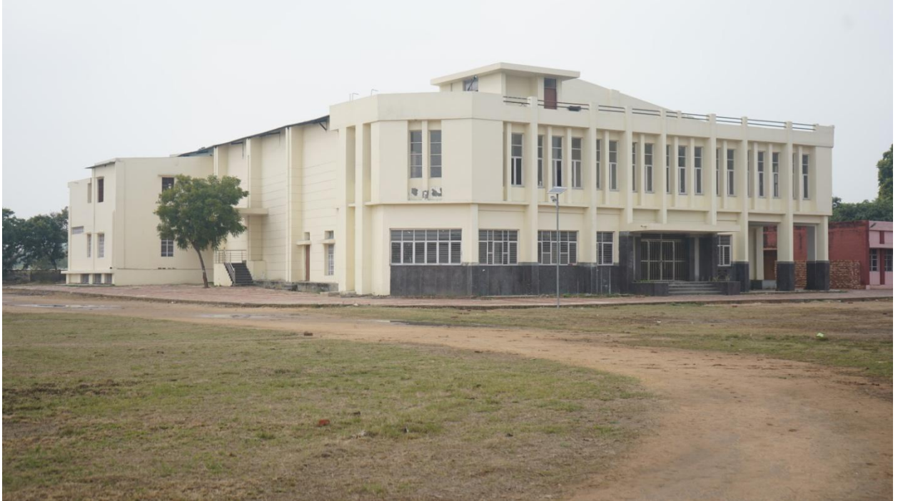
Auditorium (under construction) with a seating capacity of 600
